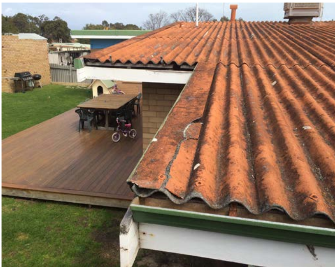
Photo 5. Part un-guttered painted ACM roof
