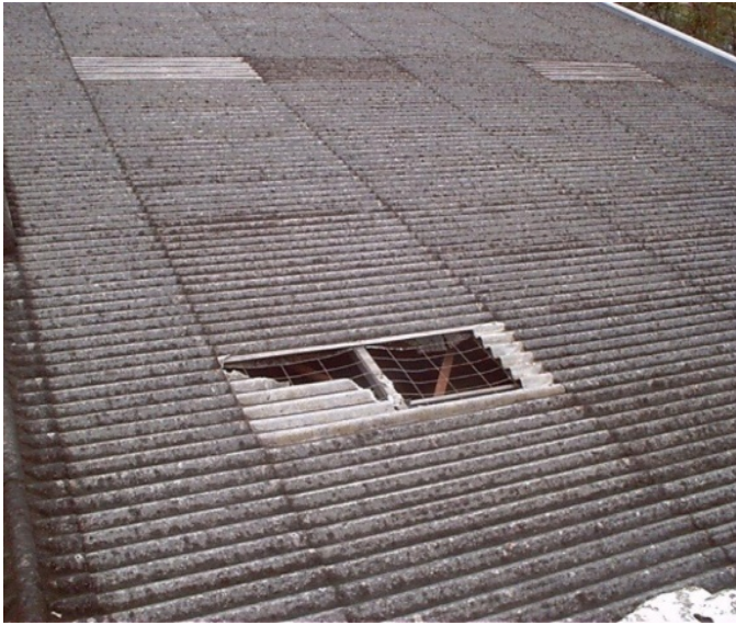
Photo 1. ACM corrugated roofing
