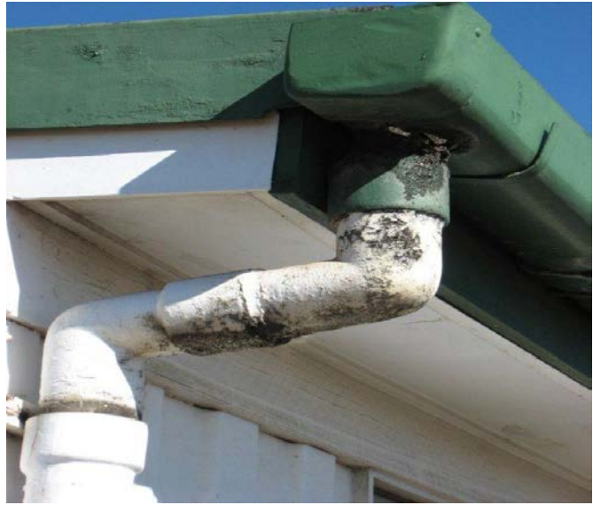
Photo 2. ACM gutter and down pipe
