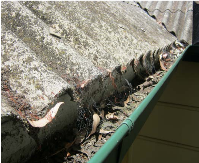
Photo 3. Asbestos fibre “whiskers” on roof lips
