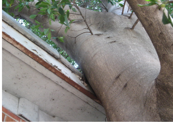
Photo 9. ACM dust settlement from sports hall roof Photo 10. Tree causing damage to ACM roof
