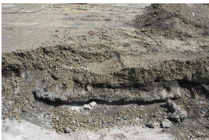
Figure 10 Buried waste FA found during site works.
